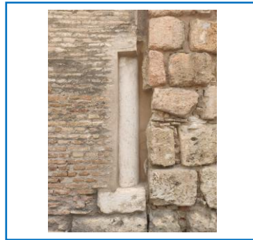
Reused column shaft in the northwest tower of the “Real Alcázar” of Seville.
